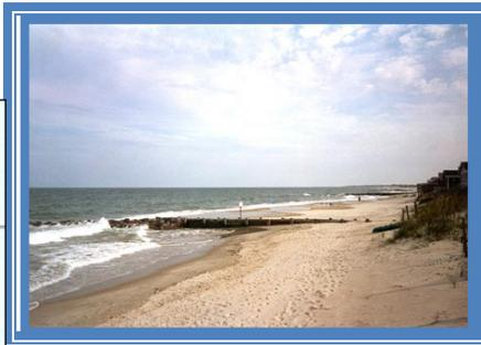
Groins are walls built perpendicular to the shoreline. They are designed to trap sand that is moving along the shore due to the long shore current. A groin usually extends to the end of the surf zone. The construction of a groin severely affects the flow of sand moved by the along shore currents, depriving down stream beaches of the sand needed for replenishment.
